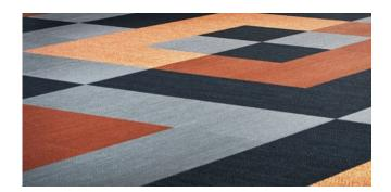
It is usual to begin installation from the middle of the room, working your way outwards. In corridors and small rooms, it may be simpler to work from one side to the other and use the centre line as a guide.
