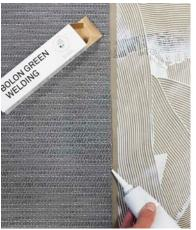
**7.** Add Bolon Green Welding along the cross-section area of the sheet. Avoid overflow on floor covering surface.
