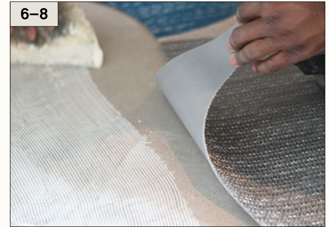
6. Finish the installation by installing the area between the reference line and the base wall. Be careful "the tongue" is sensitive and can easily be moved in horizontal direction.
